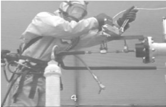
Repair work on pentaborane feed line
