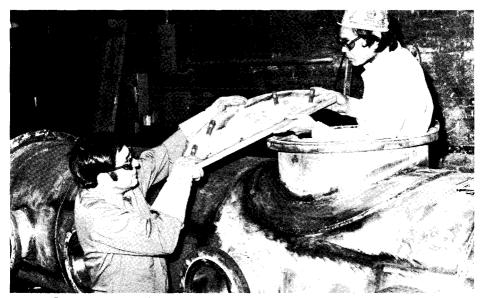
Trays are positioned prior to closing the column.
