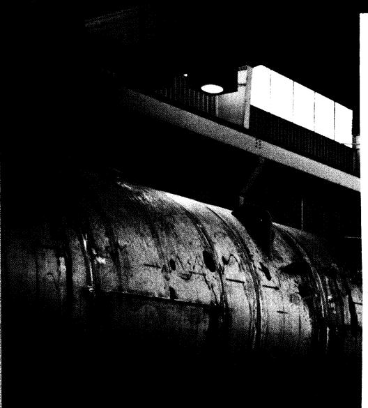
Massive 195,000 lb alcohol recovery column measuring 133' x 13½' in diameter shown leaving fabrication enroute to the job site.
