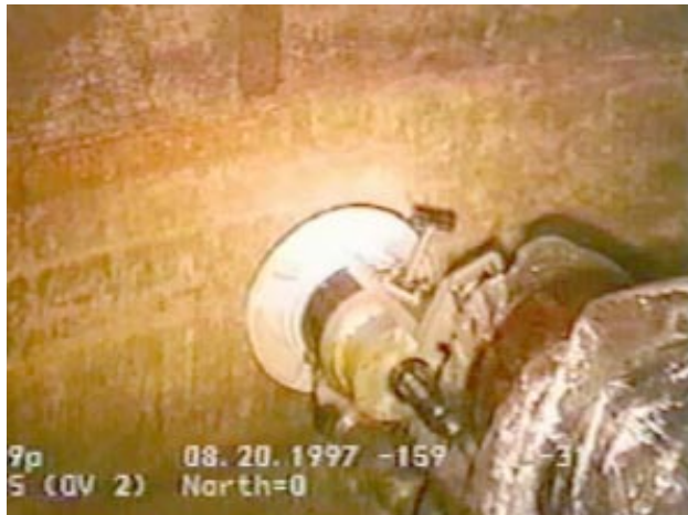
Figure 5. CSEE in position for wall scarifying.
