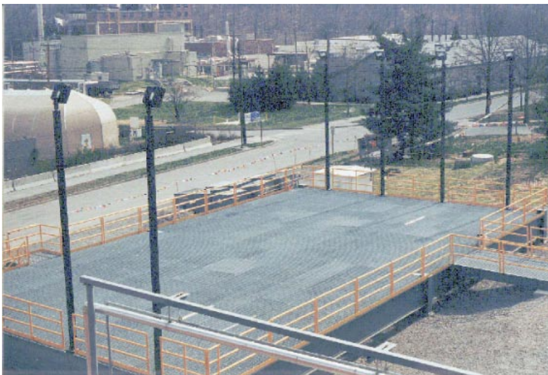
Figure 7. Load-bearing platform over Tanks W-3 and W-4.
