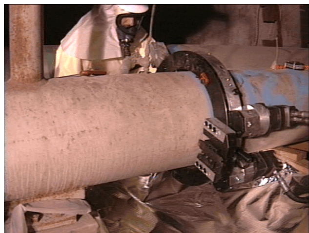
Figure 4. Setting up to cut 41-cm (16-in.) pipe.
