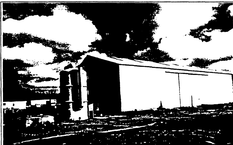
FIGURE 1: Biofilter at Augusta Fiberglass Coatings site.
