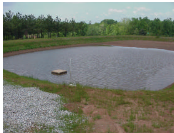
Figure 8. Photograph showing the runoff catchment. The structure in the front is the water intake.
