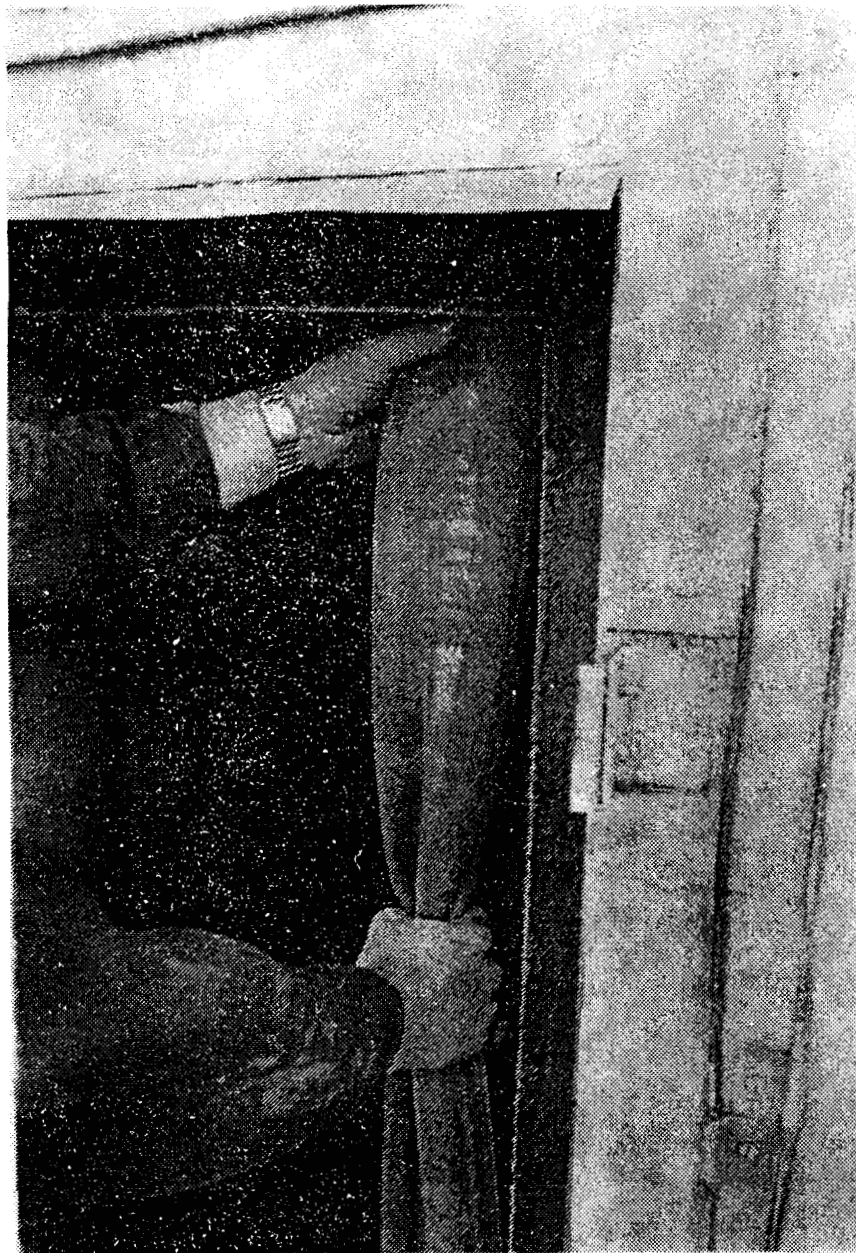
Figure 6-7. Checking for excessive build-up and poorly tensioned bags in a reverse-air fabric filter. This bag passed both tests. (Courtesy of PEI Associates, Inc.)
