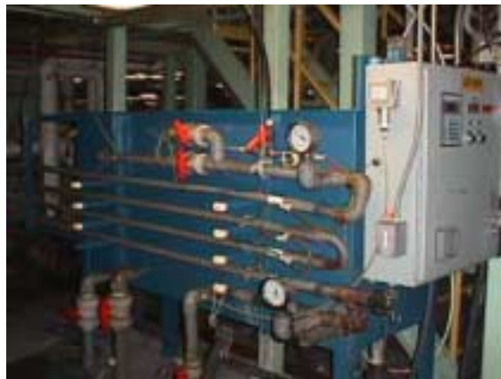
Figure 2. EWI Ultrafiltration Unit
