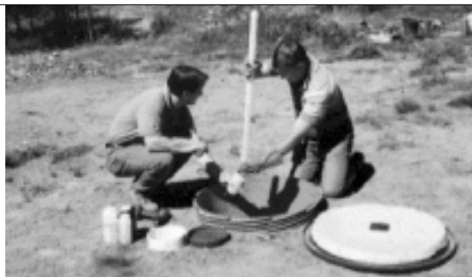
Deschutes County sanitarian Todd Cleveland and DEQ's Bob Baggett work to improve a septic system.
