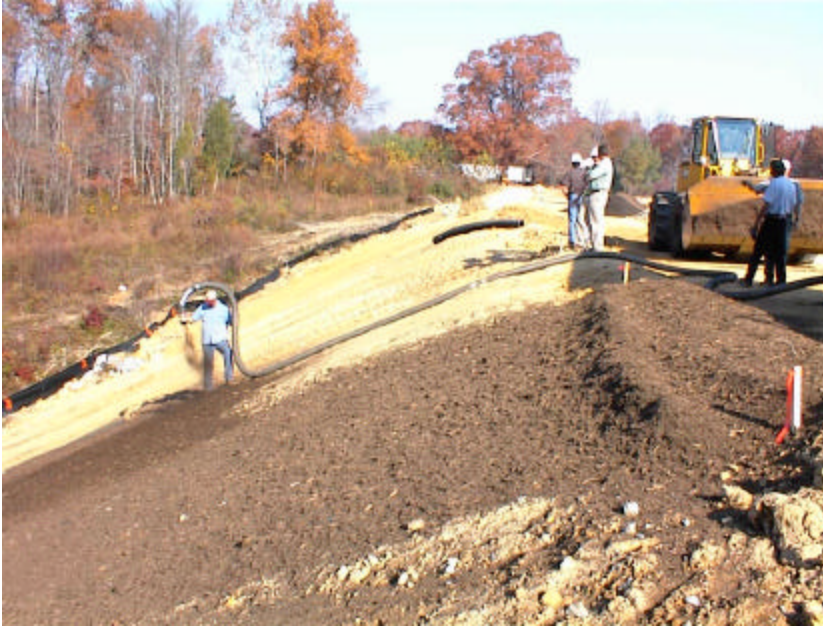
Filter berm at the top of a slope with compost
