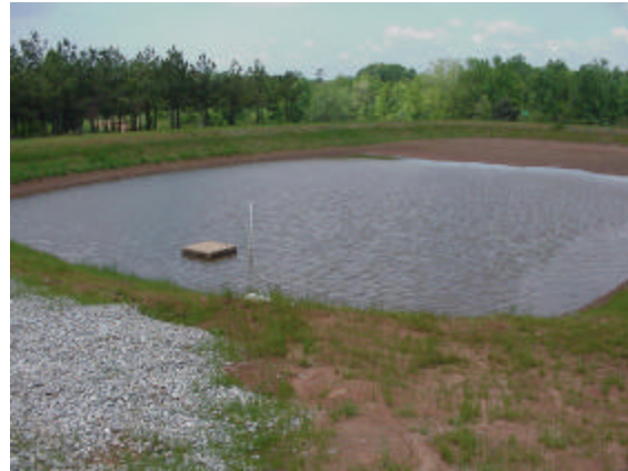
Figure 8. Photograph showing the runoff catchment. The structure in the front is the water intake.
