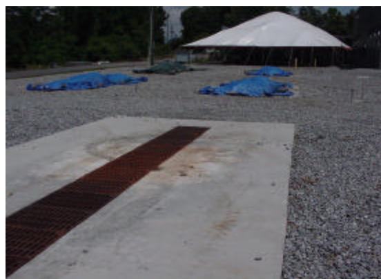
Figure 6. Concrete lined prototype windrow Pads adjacent to the research facility. The drain empties into the leachate pond (see Figure 4).
