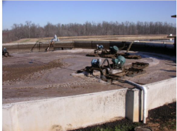
Reactor during loading and aeration
