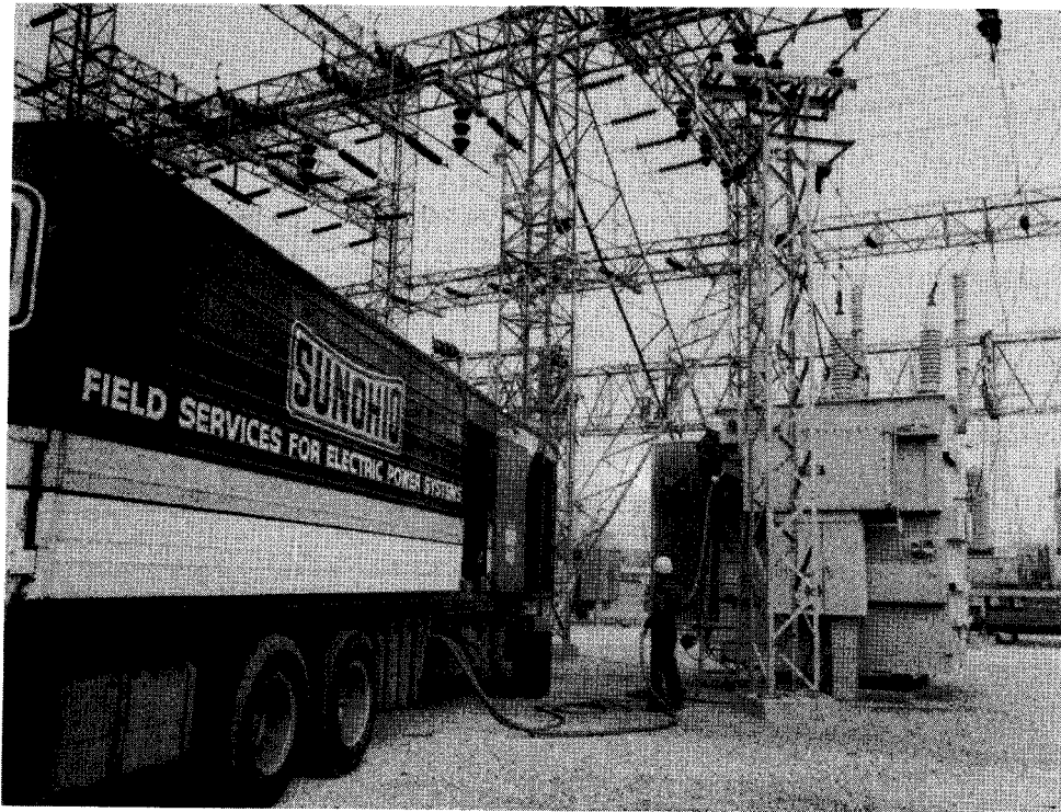
Figure 10-2 The Sunohio Treatment Unit. (a) Transformer oil is replaced without moving the transformer.
