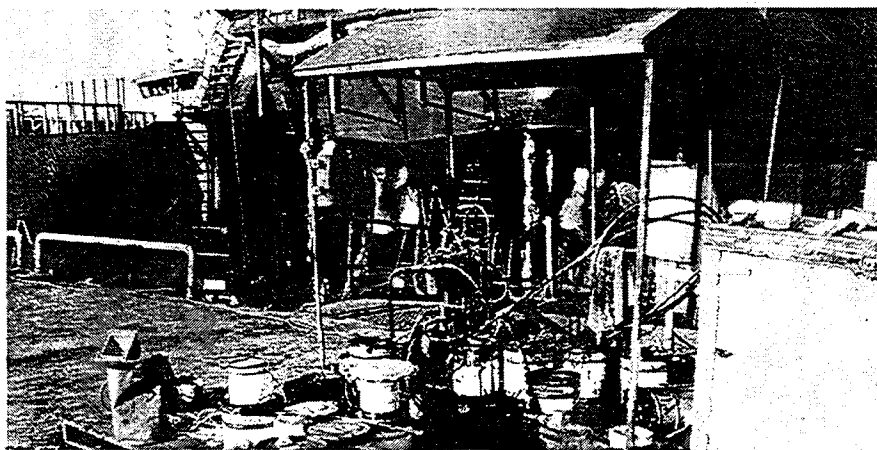
Portable shelter for paint mixing with rain cover and recessed metal floor for containment.
